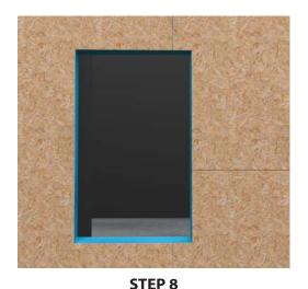
On the outside of the rough opening, over the sheathing itself, you are going to repeat the same procedure. You are going to apply a 4-inch or 6-inch wide (depending on your putty knife size) pattern of Blue Barrier Liquid Flashing 2100 around the window perimeter, so that the substrate (OSB) cannot be seen any longer, which is approximately 25 mils wet.
