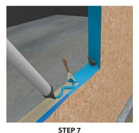
Work material into the right sill corner with your putty knife and chip brush if needed. Be sure all wood is covered. Do the same on the left and then complete the balance of the sill.
